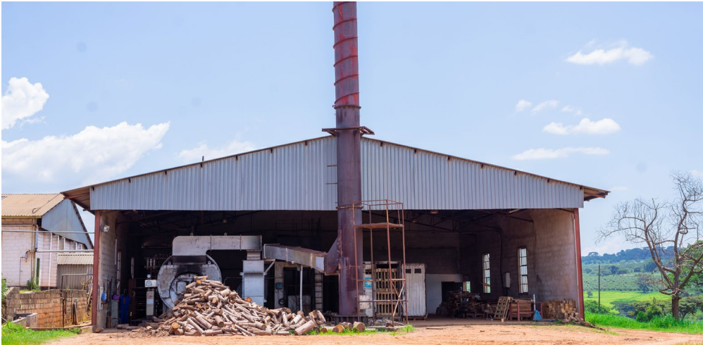
Boiler chimney on the Zona tea factory
